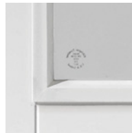
Tobago FD30 fire door has raised beading
